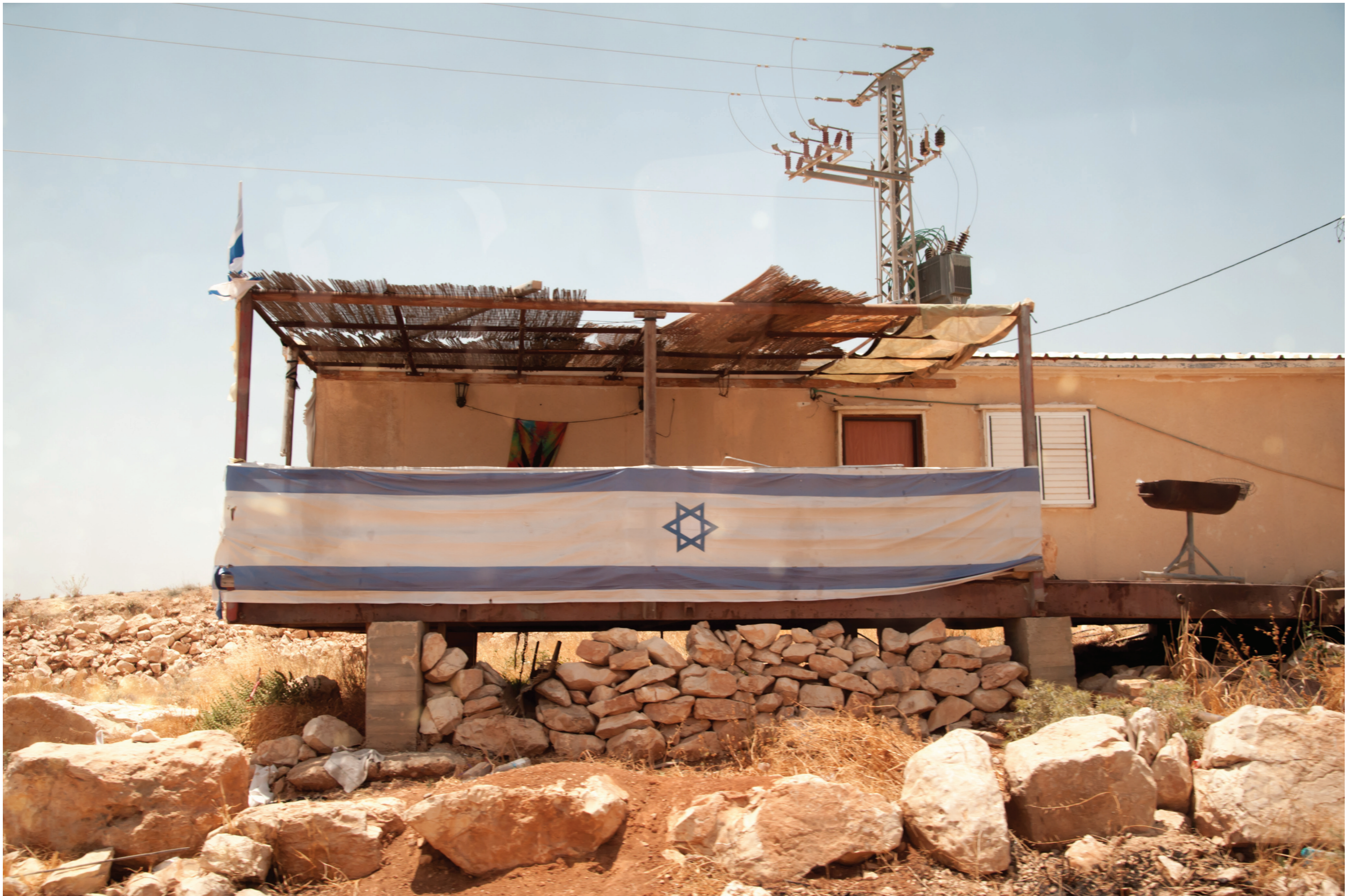
An Israeli flag hangs in the West Bank settlement outpost of Sde Bar. Built without government authorization, the outpost was retroactively legalized and connected to electricity and other utilities by the Israeli authorities. The same authorities deny access to electricity and water systems and prohibit construction of new homes in the adjacent Palestinian village of Jubbet al-Dhib.
